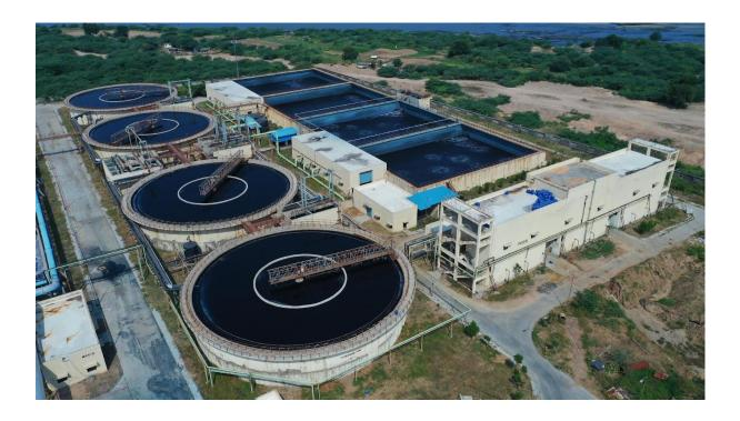
NTIEM CETP Primary Treatment in Precipitating Clarifiers. It is divided into four trains of 25 MLD each which has four equalization tanks and four primary clarifiers.
